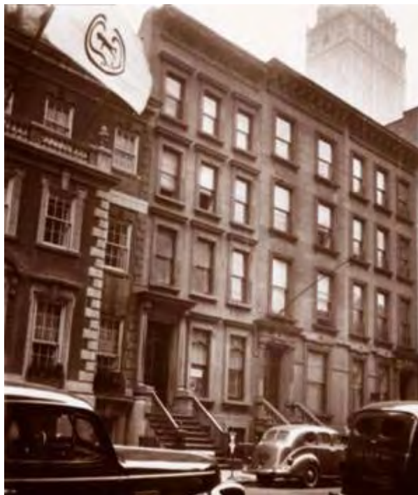
The 1880s brownstone (at center) in the early 20th century, before it became a clandestine meeting place (New York City Municipal Archives)
